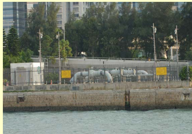
Pumping Station at Hoi Yu Street: A planning application for an expansion of the existing pumping station at Hoi Yu Street has been approved by the planning department with conditions.
