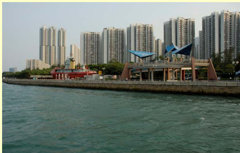
The Fireboat Alexander Grantham site aims to promote heritage appreciation, museum collection and public enjoyment. Works are in progress for completion in late 2006.
