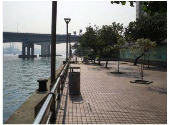
26 – Cheung Fai Road Promenade (1)
