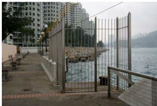
Figure 4.76: Fenced-off Landing Step in Chai Wan
