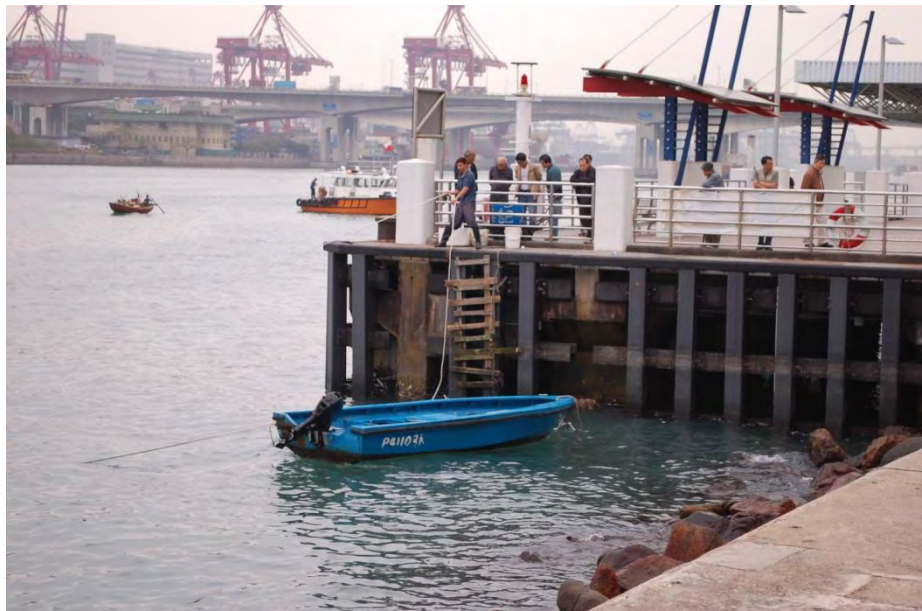
Figure 4.86: An Improvised Ladder in Tsing Yi
