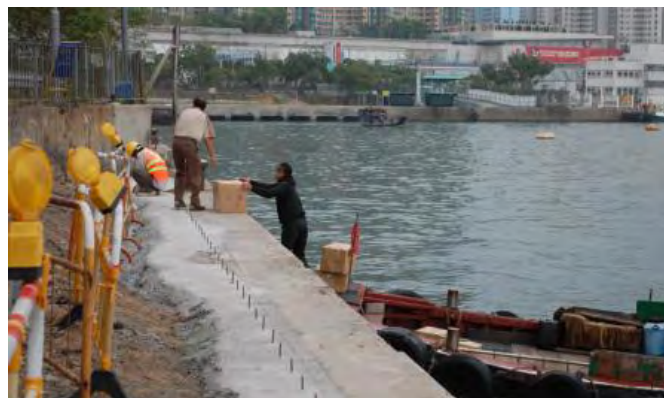
Figure 4.9: Improved Cargo-handling Area in Yau Ma Tei
