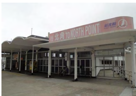
Figure 4.37: Kai Tak First Ferry Terminal
