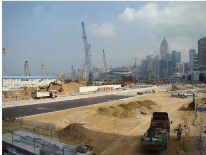
Figure 4.62: Central Reclamation Phase III
