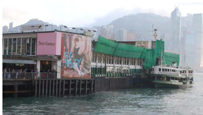
Figure 4.19: Tsim Sha Tsui East Star Ferry Terminal
