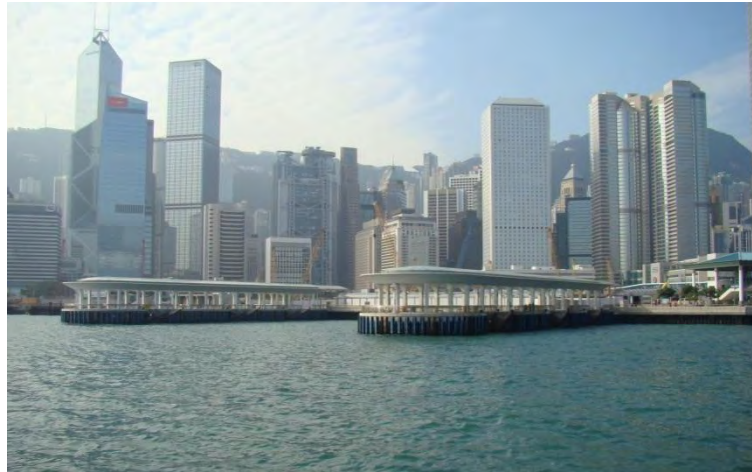
Figure 4.60: Central Piers No. 9 and 10
