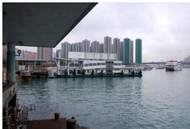
Figure 4.3: Park Island Ferry Terminal
