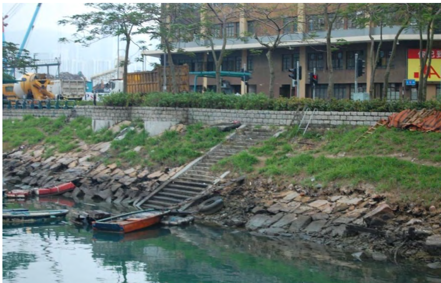
Figure 4.84: Staircase to Nowhere
