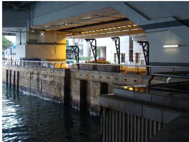
Figure 4.64: Cargo Hoists Under the Convention Centre in Wan Chai West
