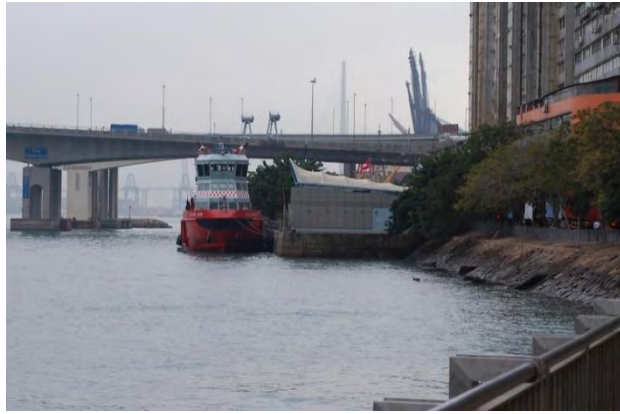
Figure 4.6: Tsing Yi Fireboat Fire Station
