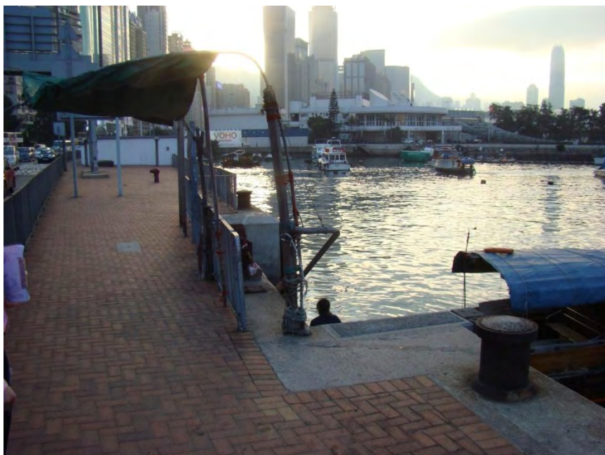
Figure 4.87: Landing Step in Causeway Bay
